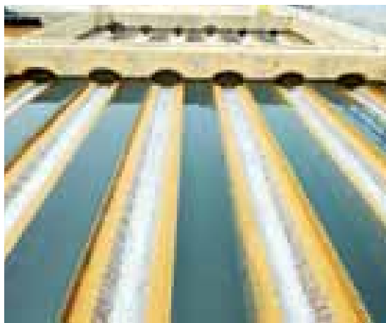
Sg Selangor Phase 2 Water Treatment Plant
