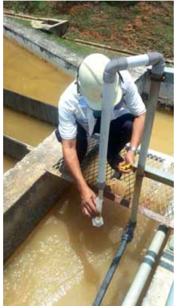
Testing of chemical dosage by WTP staff
