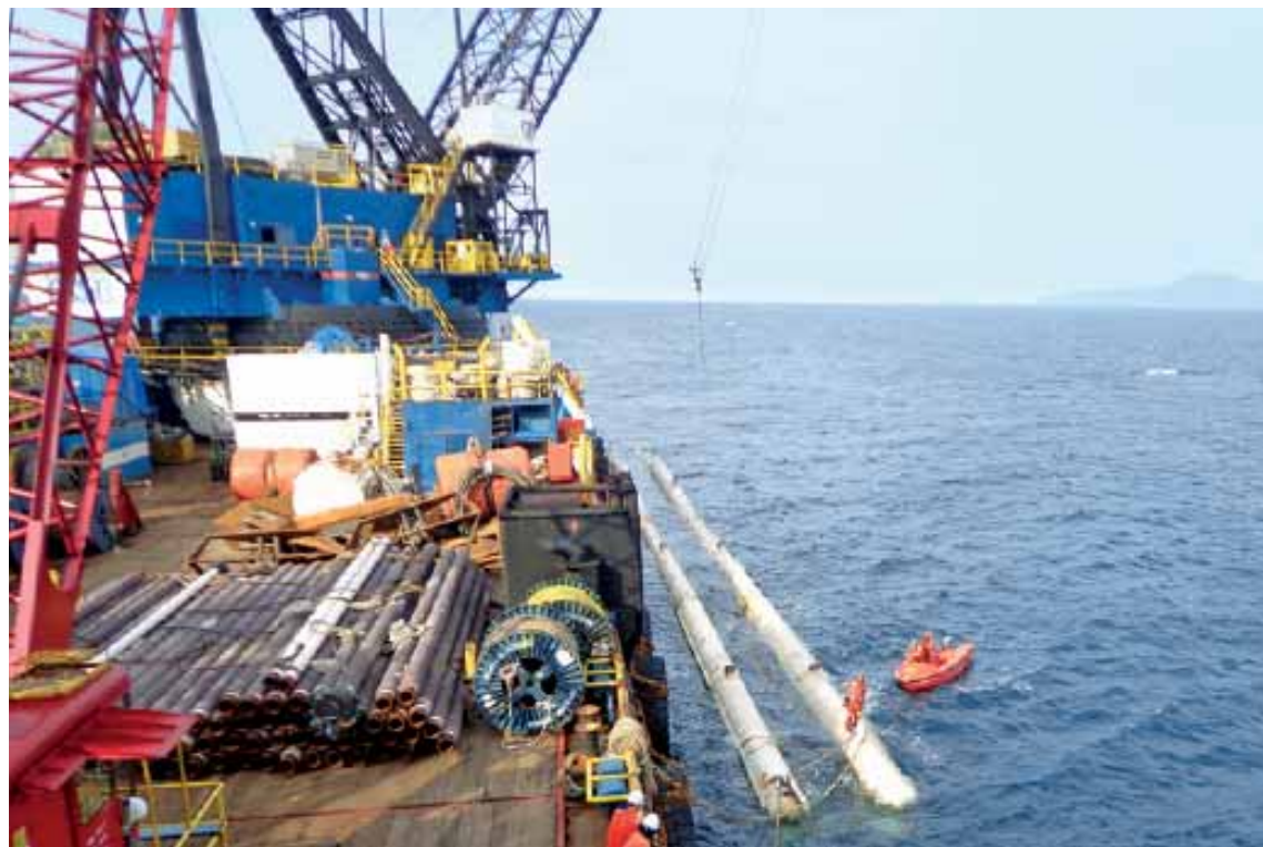
Pipe installation works in progress
