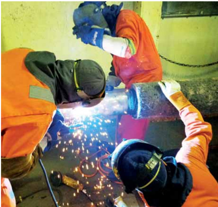
Pipe jointing works in progress
