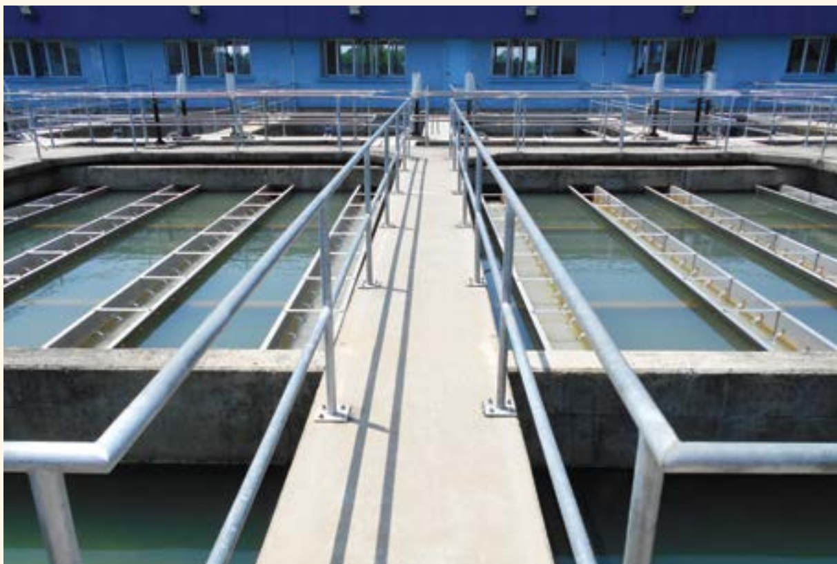
Sedimentation Tank at Kg Lawa Gadong WTP, Beaufort, Sabah
