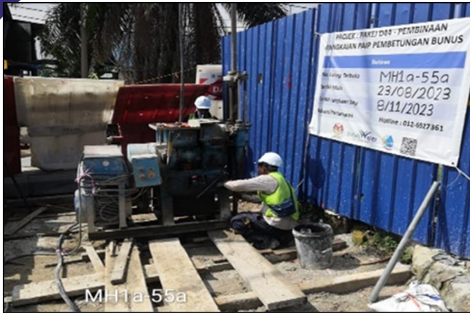
Grouting work at MH1a-55a, Zone 1a, Jalan Ayer Keroh in progress (50 of 50 points)
