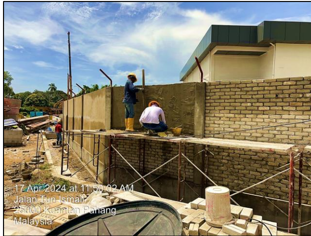
NPS 1 : Plastering brick fence in progress
