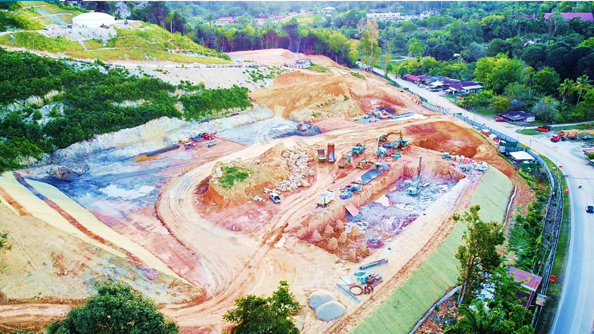
EARTHWORK & PILING WORKS AT WATER TREATMENT PLANT
