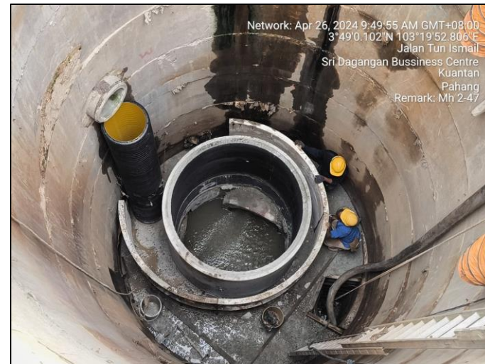
Zon 2: Construction of pit for MH2-47 in progress
