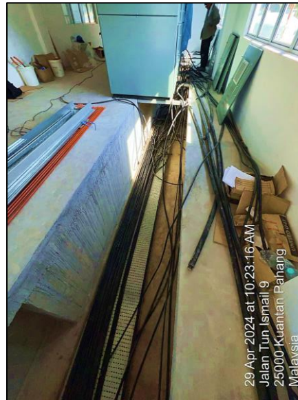
NPS 1 : electric cable installation in progress
