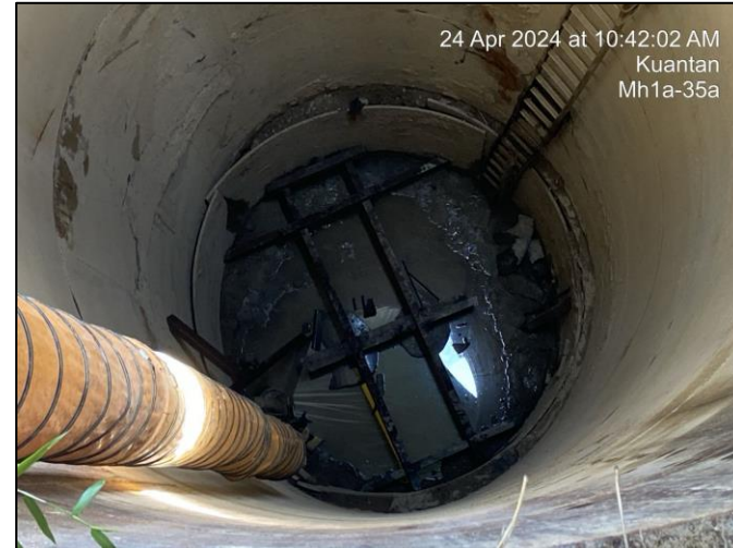
Zon 1: Preparation for pipe jacking work from MH1a-35a to MH1a-35
