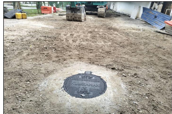
Manhole at MH3-1c, Zone 3, Jalan L5 completed
