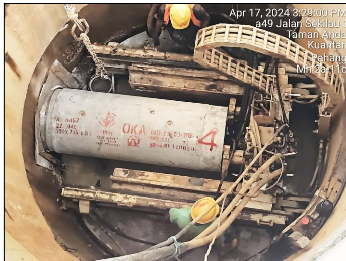
Zon 2: pipe jacking work from MH2a-11C to MH2a-11B in progress
