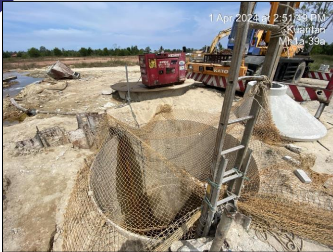
Zon 1: Construction of pit for MH1a-39a in progress
